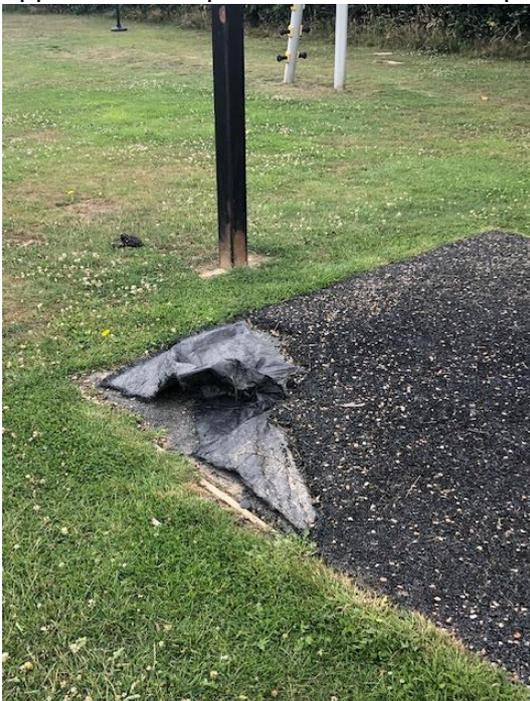
**Resolved: To contact the company who installed the play equipment as the surface should not have lifted at the corner.**
